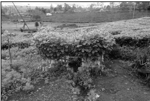
Soakage pits for waste water - Mattakekke Estate
