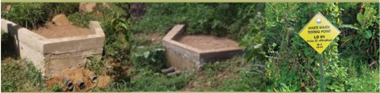
Filtration through Concrete Bunds (rock, gravel, sand) and Biological Filtering
