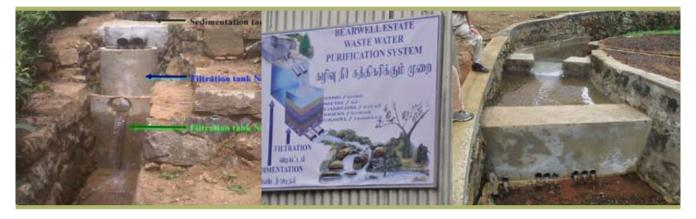
Sedimentation and Twin Filtration (rock, gravel, sand) through Concrete Cylinders
