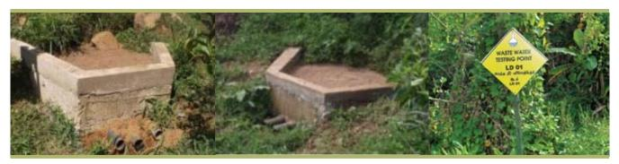
Filtration through Concrete Bunds (rock, gravel, sand) and Biological Filtering
