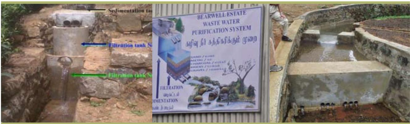
Sedimentation and Twin Filtration (rock, gravel, sand) through Concrete Cylinders - Great Western Estate
