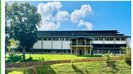
New factory building followed green building concept
