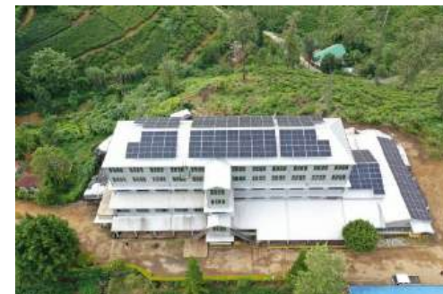
Rooftop Solar Generation
