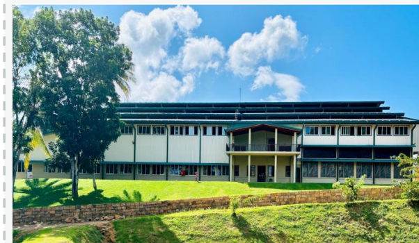
New factory building followed green building concept
