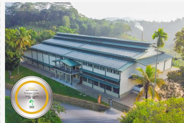
Kiruwanaganga Green Factory / renewable energy
